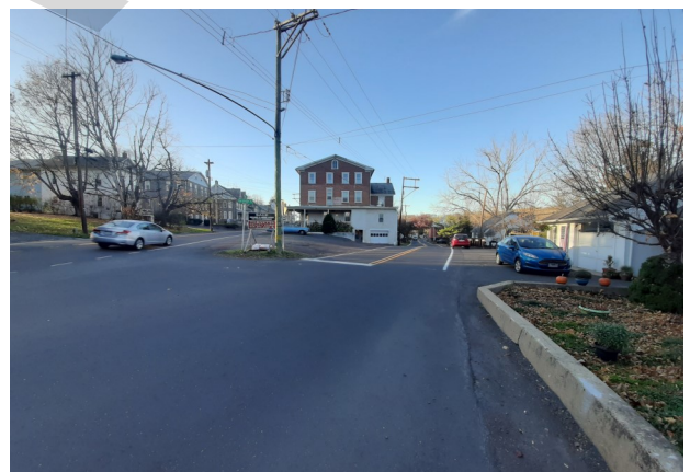
Poor Intersection Design of Geryville Pike and Sumneytown Pike
