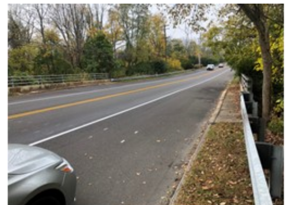
Flooding Location over Haines-Dittingers Creek
