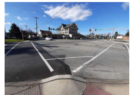
Pedestrian crossings at Skippack Pike, Whitpain Township
