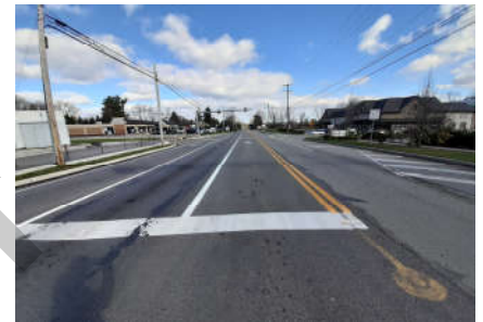
Closely Spaced Commercial Driveways Near the Intersection of Butler Pike and Skippack Pike
