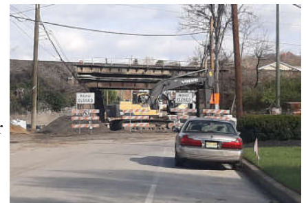
Sinkhole Remediation Project on Butler Pike
