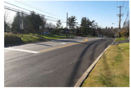
Closely Spaced / Skewed Intersection of Germantown Pike with Sunset Avenue / Sandra Lane
