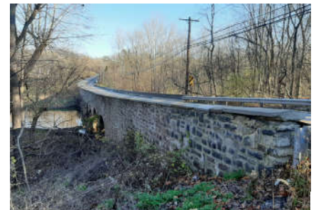
Stone Arch Bridge over Skippack Creek
