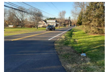
Aboveground Utilities, Marlborough Township
