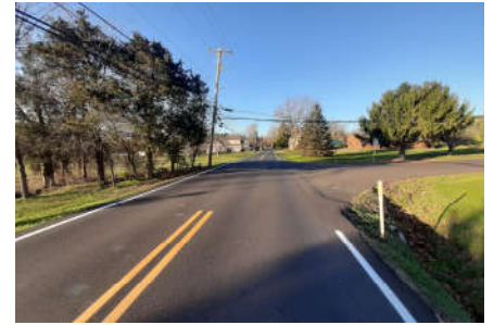
Drainage swale along edge of roadway, Marlborough Township
