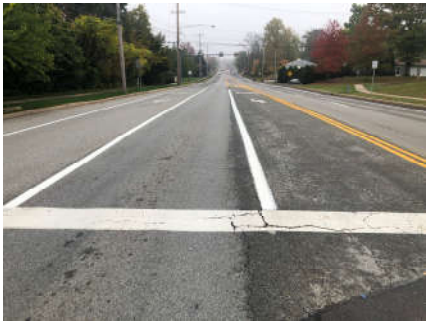
Lane drop at Suplee Road, Upper Gwynedd Township
