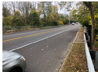
Flooding location over Haines-Dittingers Creek
