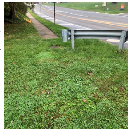
Sidewalk abruptly stopping along Sumneytown Pike, Upper Gwynedd Township
