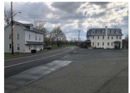
Utilities and buildings near edge of roadway, New Hanover Township
