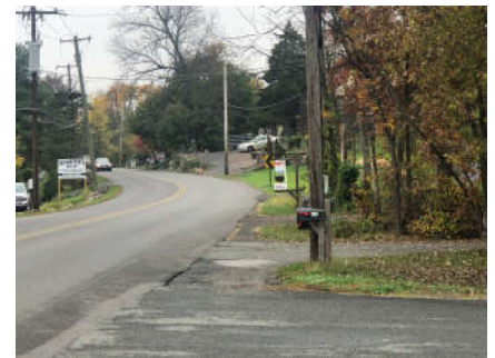
Utility poles near road make widening difficult to achieve
