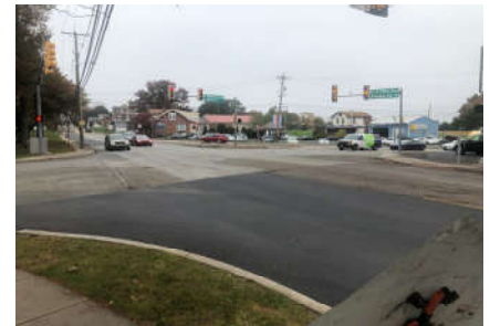
Intersection at Gilbertsville Road
