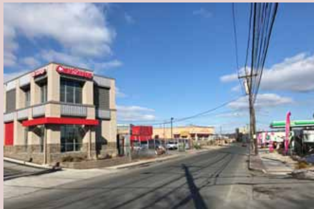
Existing conditions along South Columbus Avenue include wide travel lines, a lack of street paint, narrow sidewalks, and no street trees.
