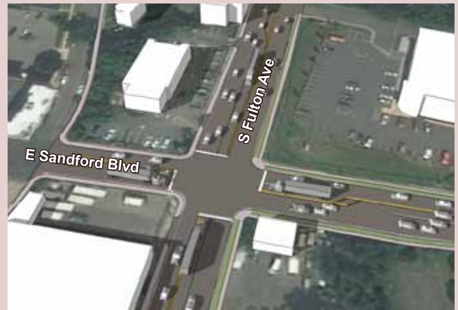
Existing conditions at this intersection.
