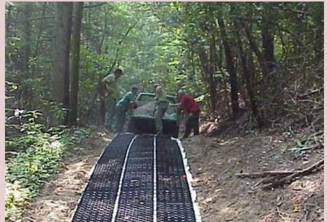
Lining the pedestrian and bike paths with geotextiles or permeable pavers will improve the sediment controls throughout the Hutchinson River Parkway Trail.
