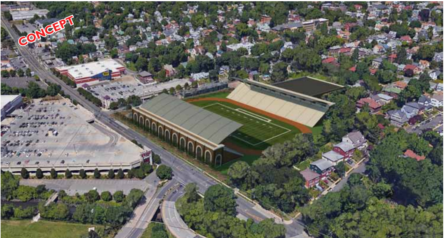
A one-tiered seating system on both sides of the track allows for more capacity while keeping the height of the grandstand low. A low parking requirement makes a small parking structure possible.
