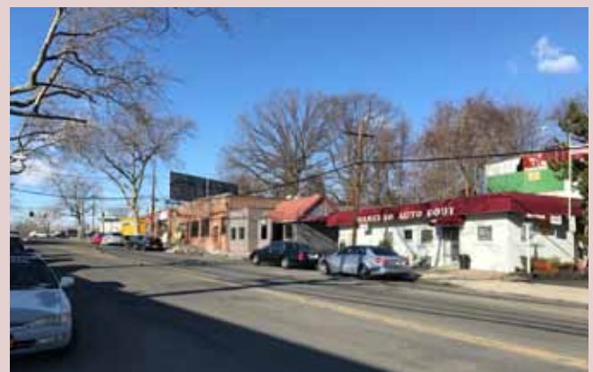
Existing conditions looking north on South Fulton Avenue toward the intersection of East Sanford Boulevard.
