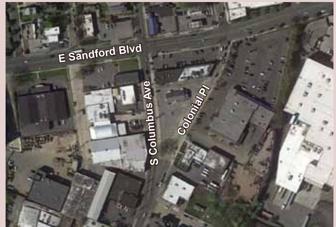
Existing conditions at this intersection include large amounts of parking lots, narrow sidewalks, wide lanes, and very few street trees.
