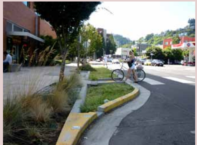
Green infrastructure divert, or capture and treat roadway runoff before discharging into the Hutchinson River.
