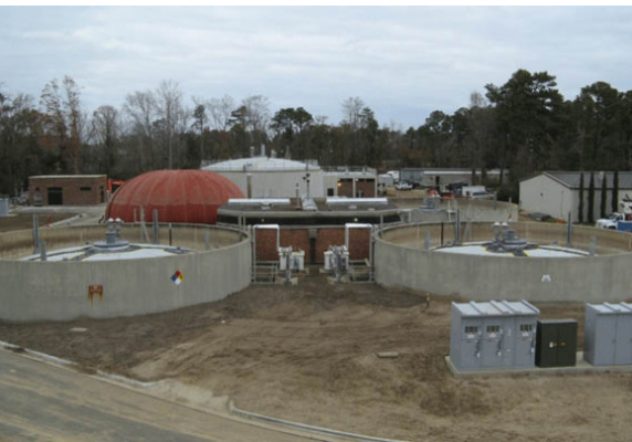
Northside Wastewater Treatment Plant The Northside Wastewater Treatment Plant was originally put into service in 1970 as an 8,000,000-gallon per day treatment facility. After a $80,000,000 upgrade in 2009, the plant now has a 16,000,000-gallon per day treatment capacity.
