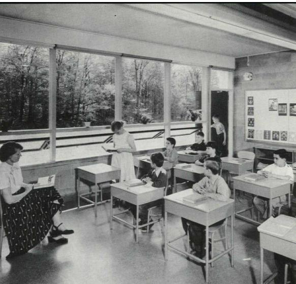
From each of the classrooms (above), a door opens to the outside. Sash, combining fixed panels and pivoting units, are of wood. For acoustical control, ceilings are finished in random-perforated cane-fiber tile. Artificial lighting is from 8-ft, surface-mounted fluorescent fixtures.
