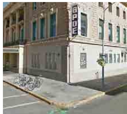
The northeast corner of the intersection of Front Street and Pattee Street lacks curb ramps for access from the street to the sidewalk
