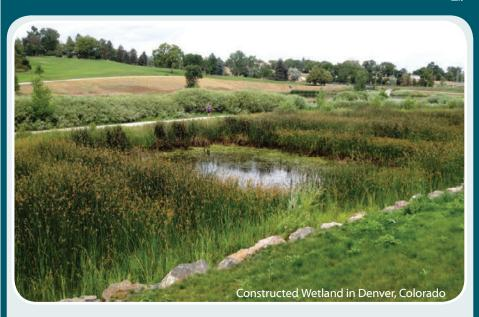
Stormwater Best Management Practices are critical in constructed environments to filter and manage stormwater runoff within developed areas. Examples include green streets, bioswales, pervious pavements, rain gardens, large constructed wetlands, and green roofs. There are many functional benefits to these techniques including reduction of erosion, thermal and chemical pollution, lose of habitat and wildlife, etc.
